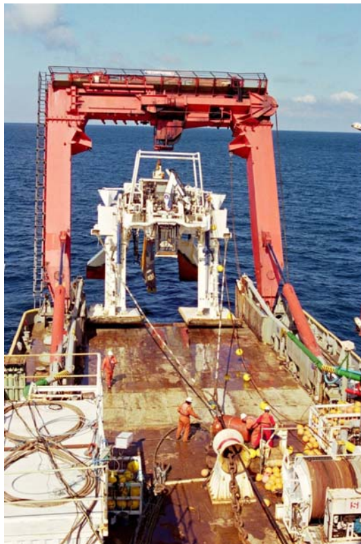
Figure 4-F : Modular Cable Plough in use on Isle of Man interconnector
